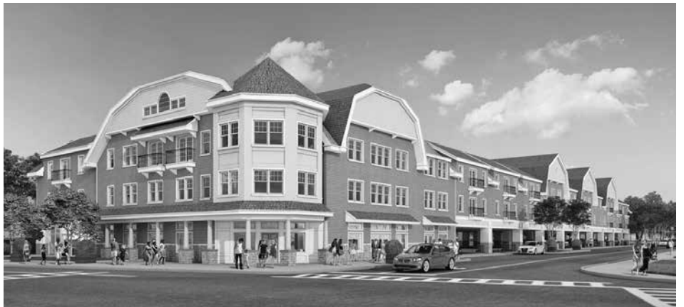
The Grove housing complex has been announced by the Northwind Group at the corner of Grove Avenue and East Main Street on the East Patchogue-Patchogue line. The proposed 80,000-square-foot structure would consist of 80 residential units on the second and third stories and retail on the first floor, facing the street.
